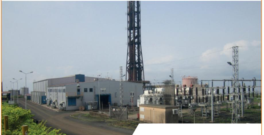
**ENEO CAMEROON'S** Limbe power plant could generate only about 40% of the installed total capacity of 80MW. Wärtsilä's solution was a complete rehabilitation; a total overhaul of four Wärtsilä engines and five alternators. The overhaul covered all critical auxiliaries, including the replacement and upgrade of radiator systems as well as other auxiliaries.
