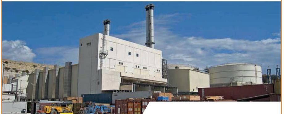
**SHANGHAI ELECTRIC POWER**, one of the major listed companies of China Power Investment Corporation, reduced both electricity production costs and emission levels at their Delimara 3 Power Plant in Malta. Eight Wärtsilä HFO-fuelled engines were converted to run on natural gas and a new UNIC C3 engine control system was installed.
