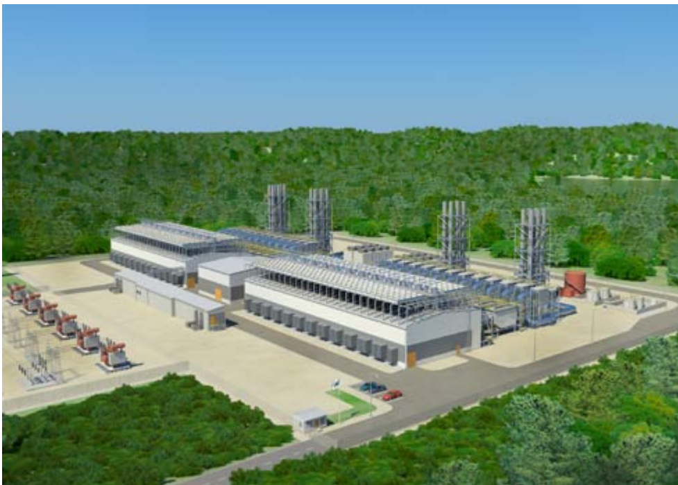
A 500 MW Flexicycle™ power plant based on 24 Wärtsilä 18V50SG units in combined cycle.
