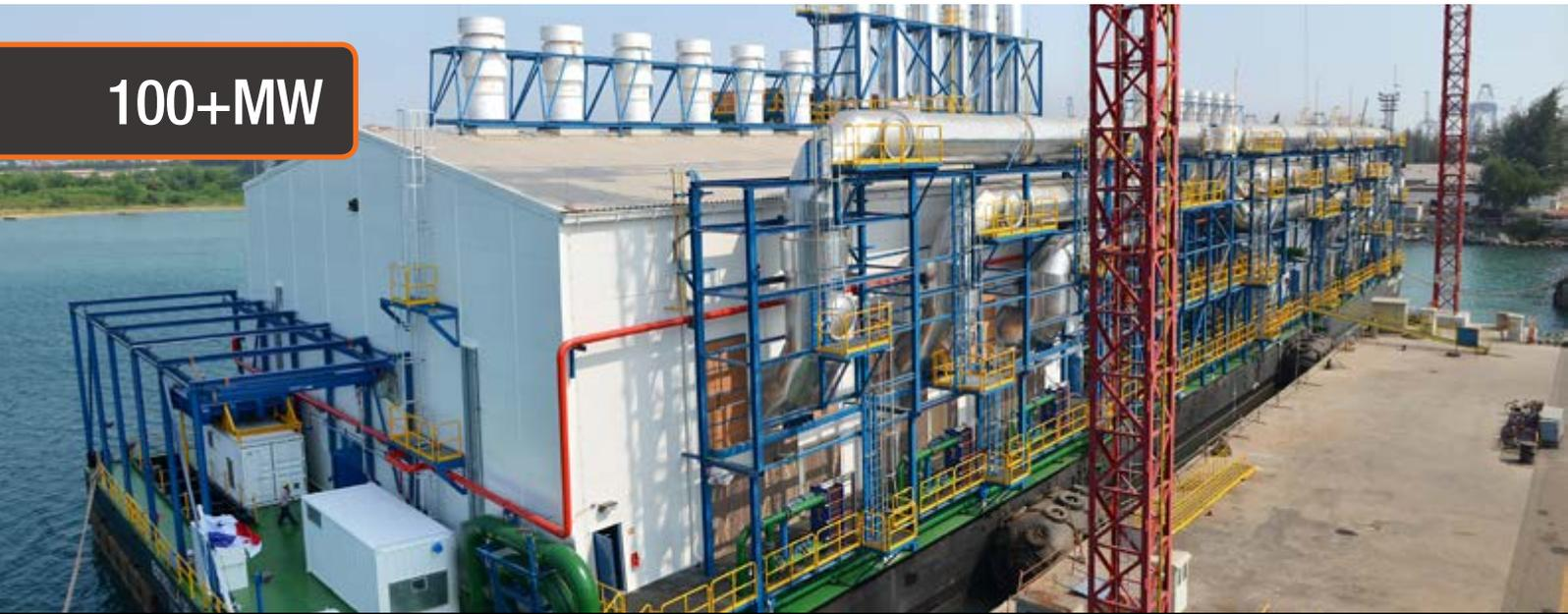
Seaboard Flexicycle power plant, Dominican Republic, with 6 x Wärtsilä 18V50DF engines providing a total output of 110 MW.
