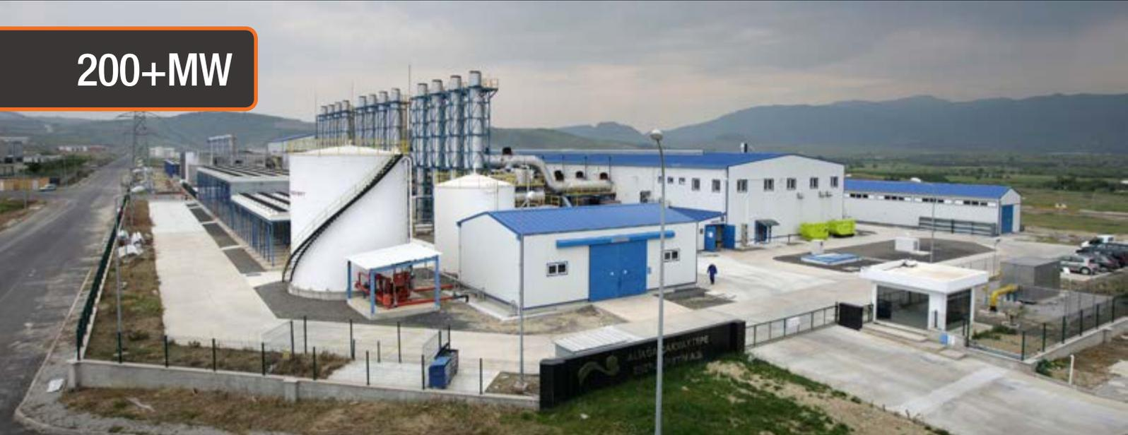
Aliaga Flexicycle power plant, Turkey, with 28 x Wärtsilä 20V34SG engines providing a total output 270 MW.
