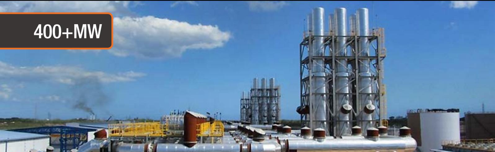
Quisqueya I & II Flexicycle power plant, Dominican Republic, with 2 x 12 x Wärtsilä 18V50DF engines providing a total output of 430 MW.
