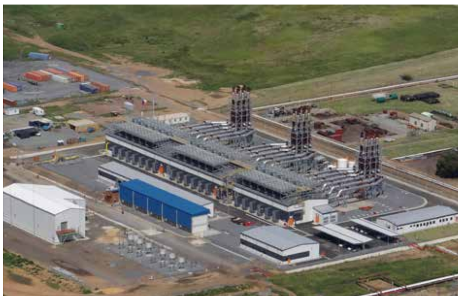
The Sasolburg power plant in South Africa.
